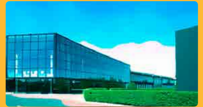
Under construction Building Qom High Way | Tehran | 4(Km) After Tax Road
